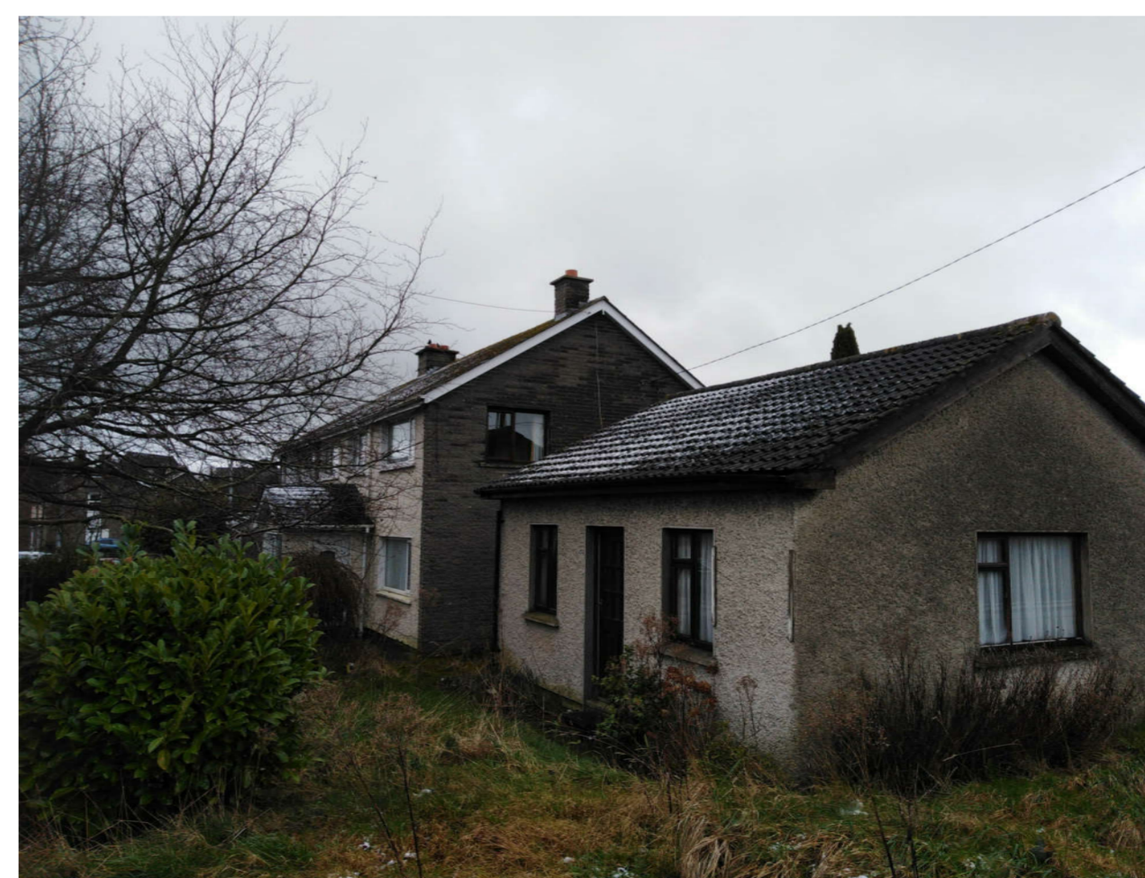
IMAGE 3. EXISTING SINGLE STOREY STRUCTURE TO BE DEMOLISHED
